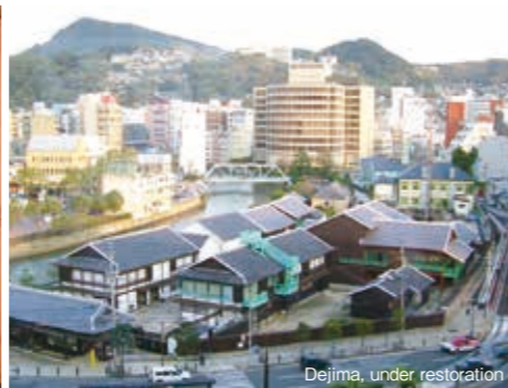
Dejima, under restoration
