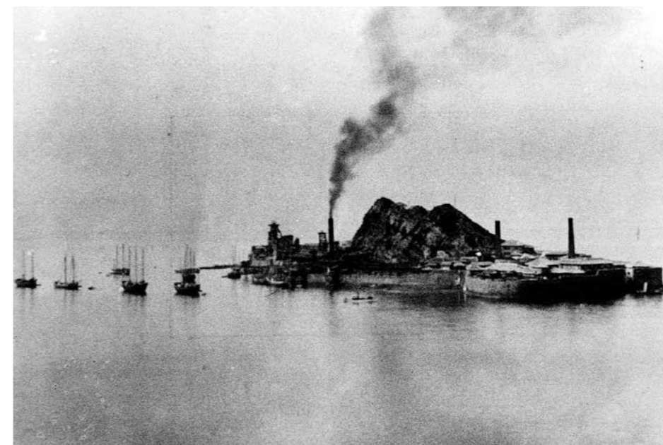
A tunnel spewing smoke. 1901 ("Hashima (Gunkanjima)," Takashima Board of Education)
